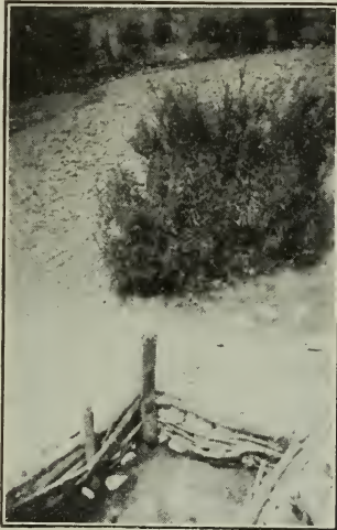
FIG. 108.—Well with wattle walls sunk in sandy bank of stream.
